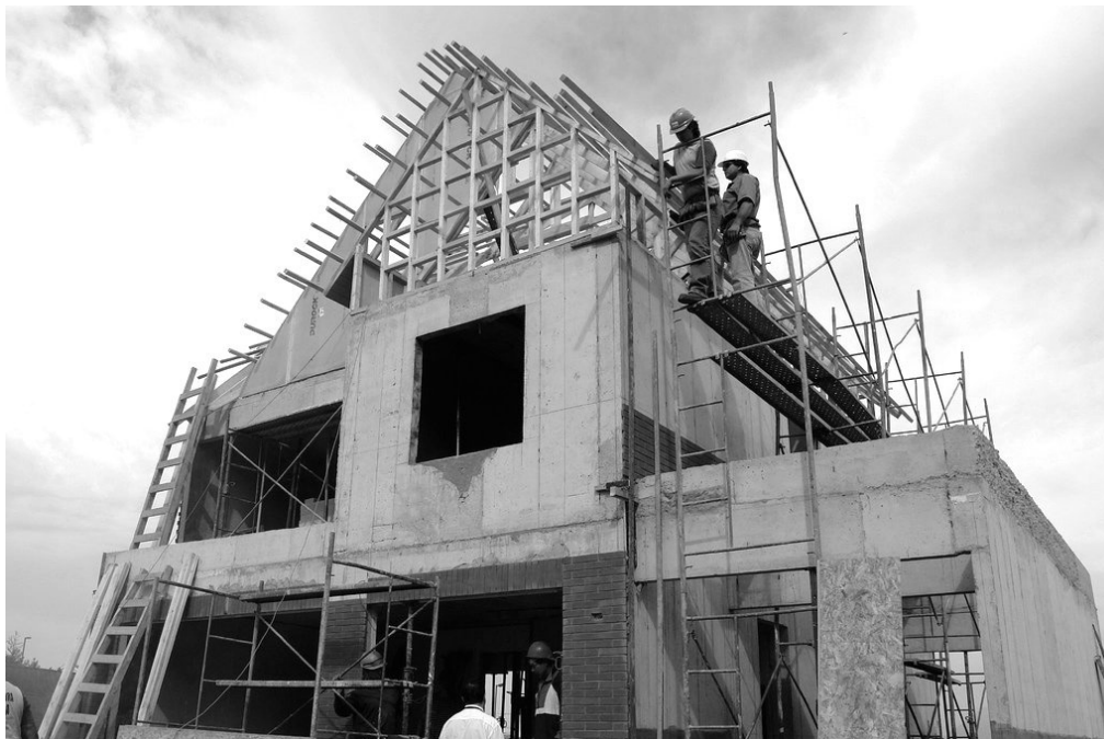
Photo: concrete forms
